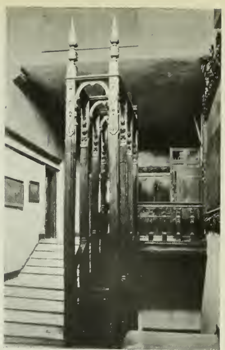
SAFFRON WALDEN. (3). Audley End, early 17th-century, Head of S. Staircase.
